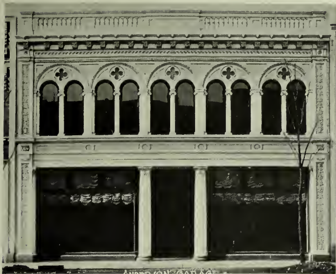
ANDERSON GARAGE, CHICAGO, ILL.
